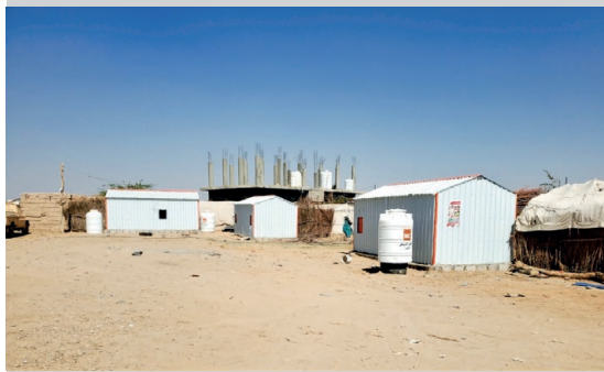
NRC handed housing units for IDPs.
