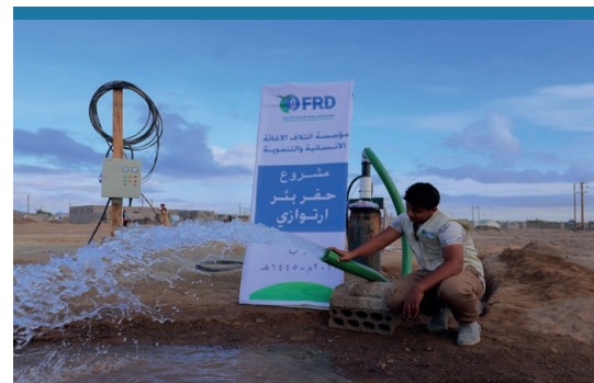
FRD - Artesian Well Drilling Project.
