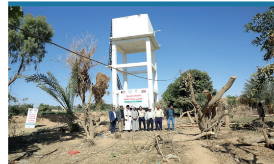
SCRD - water tank construction.
